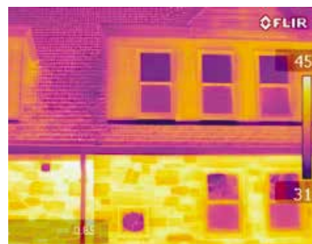
Figure 7. Exterior infrared image of a dormitory building at a college in Philadelphia, Pennsylvania, originally built 1981.
