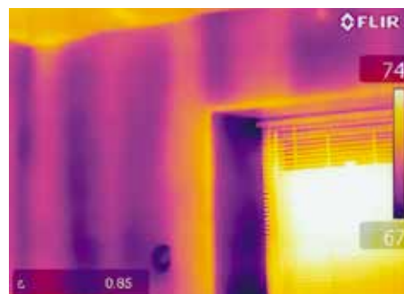
Figure 10. Interior infrared image of a historic home and office at a college in Philadelphia, Pennsylvania, originally built 1724.
