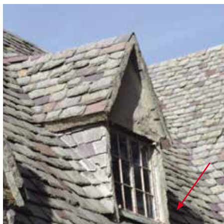
Figure 3. Install sensors on the north slope under shade (wintertime); red arrow indicates the sensor location.
