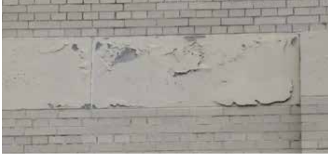
Figure 4. Cast stone units at the belt course with blistered and peeling coatings and efflorescence. The top and bottom photos are from 2015 and 2019, respectively.
