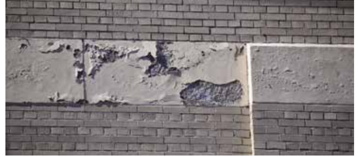
Figure 4. Cast stone units at the belt course with blistered and peeling coatings and efflorescence. The top and bottom photos are from 2015 and 2019, respectively.
