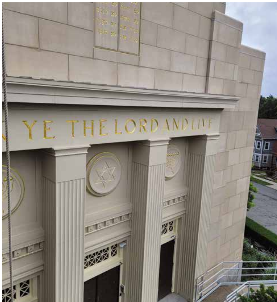
Figure 8. The restored Temple Emanu-El with new cast stone units, a glass-fiber-reinforced polymer cornice, and gilding completed.
