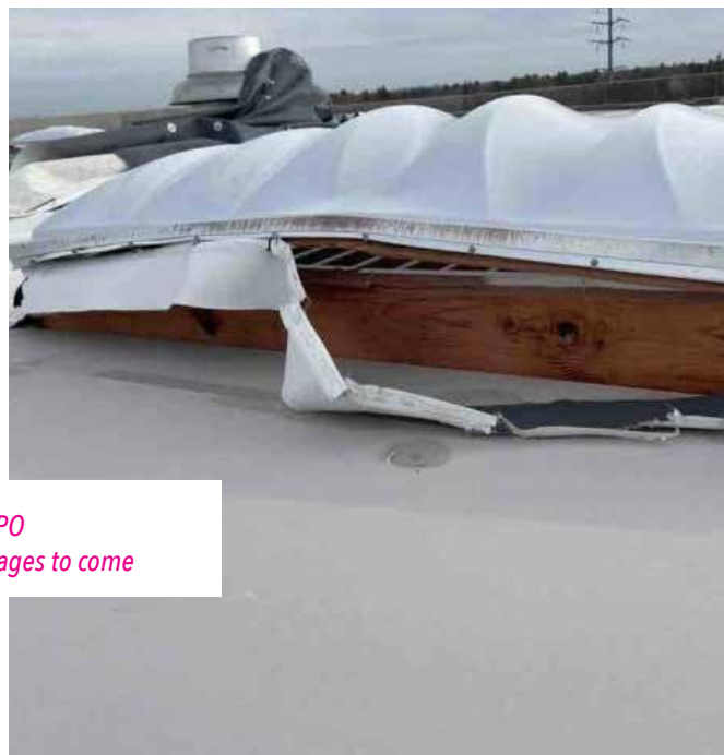
FIGURE 2. Curb and skylight separation from the deck.
