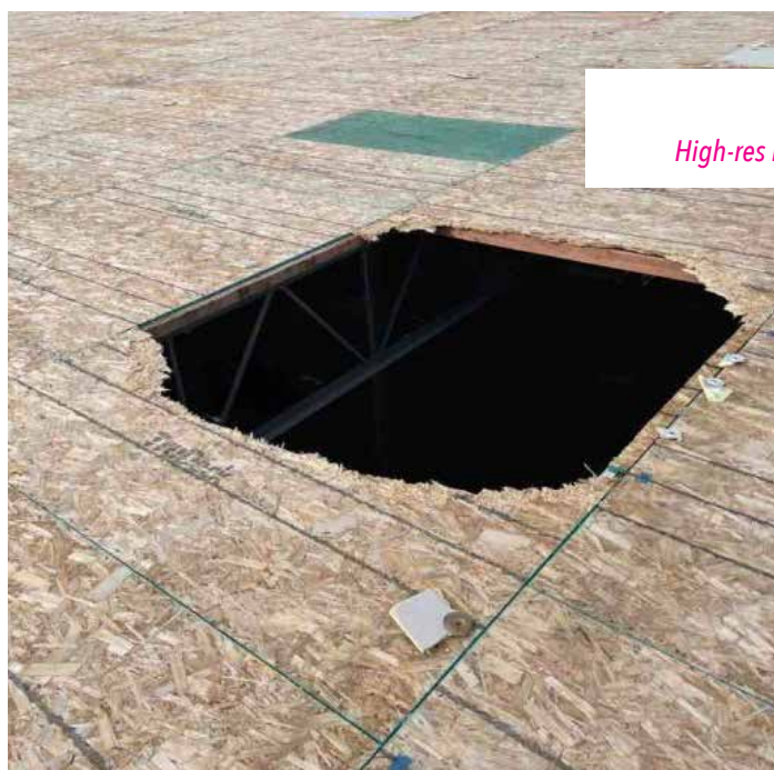
FIGURE 3. Loss of rooftop curb due to possible internal pressurization.
