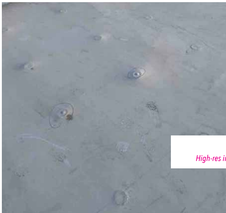
FIGURE 1. Extensive fastener withdrawal with no corresponding wind event.
