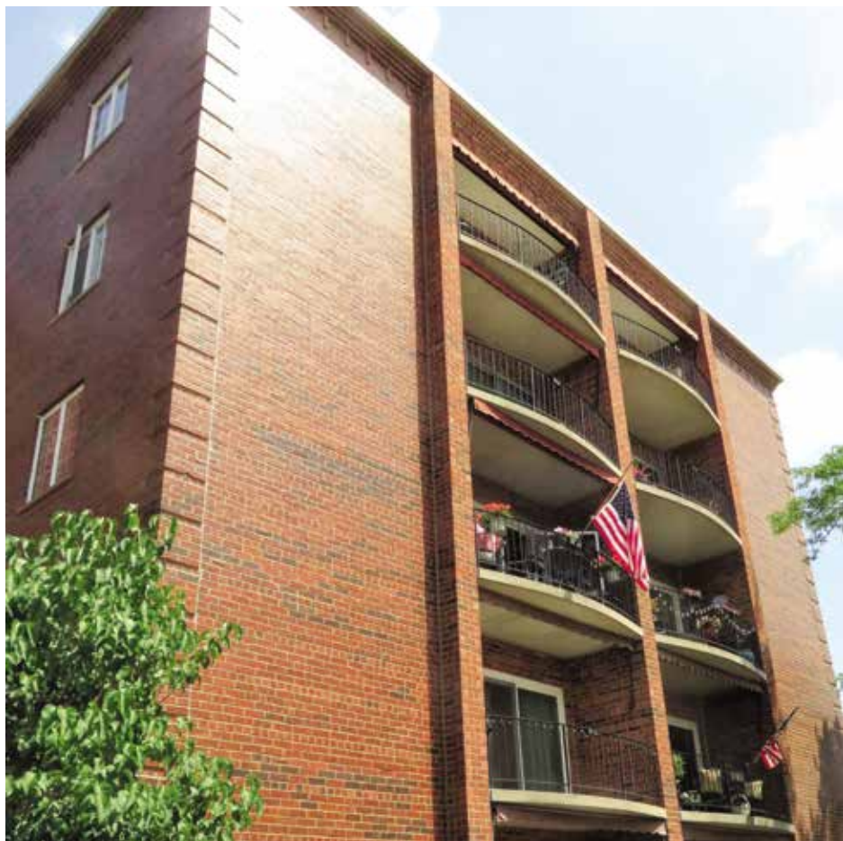
Figure 15. Translucent silicone coating applied to the exterior face of a two-wythe mass masonry wall.
