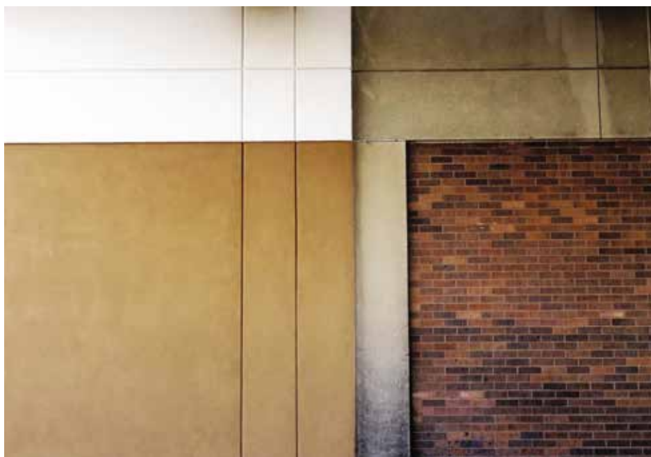
Figure 12. Completed overclad area of the EIFS adjacent to the existing masonry exterior wall.
