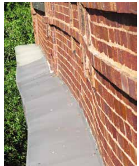
Figure 4. Two examples of masonry wall bowing due to lack of movement joints.
