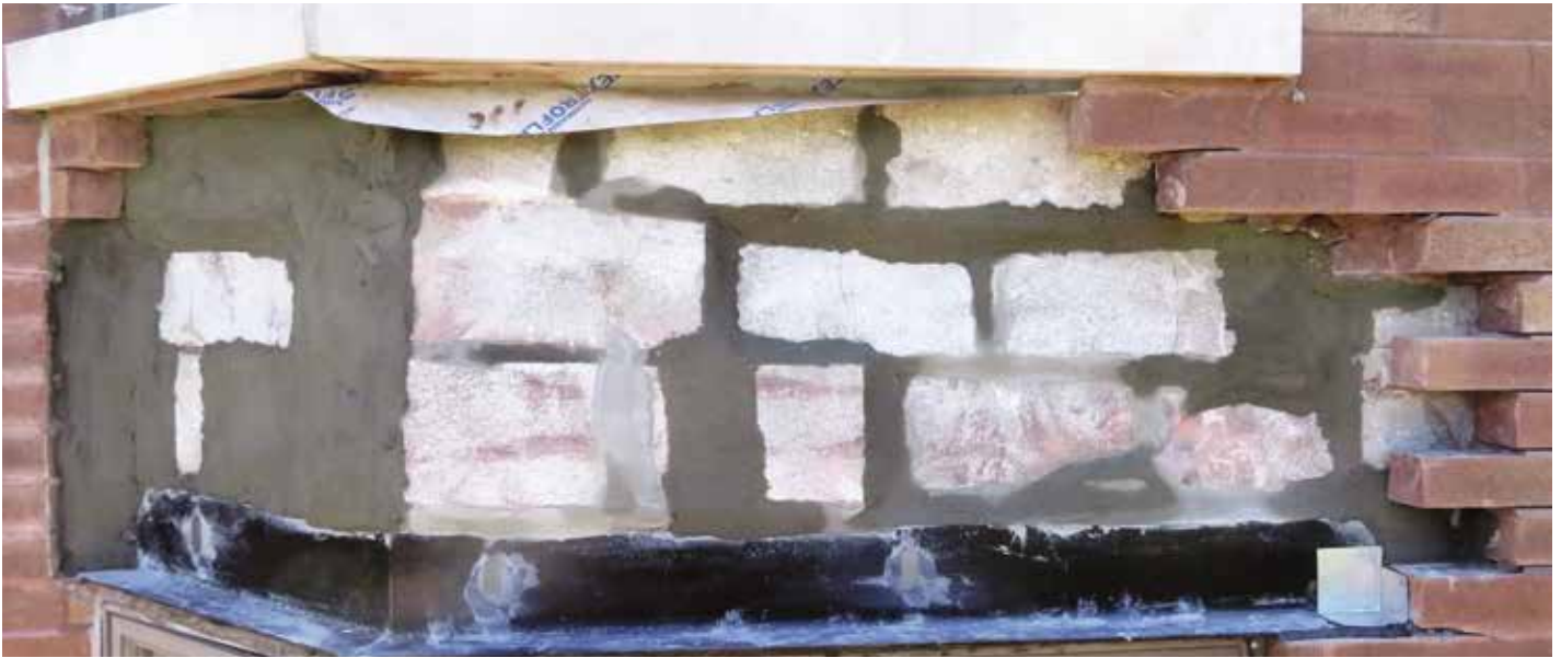
Figure 9. Preparation of a backup wall prior to installation of the AWB and through-wall flashing.
