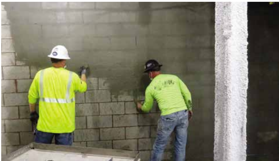
Figure 14. Crystalline waterproofing application on the interior side of a CMU wall.
