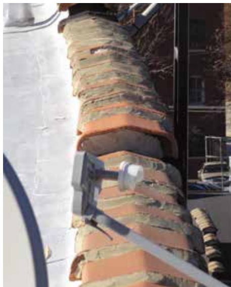
Figure 4. Two examples of masonry wall bowing due to lack of movement joints.
