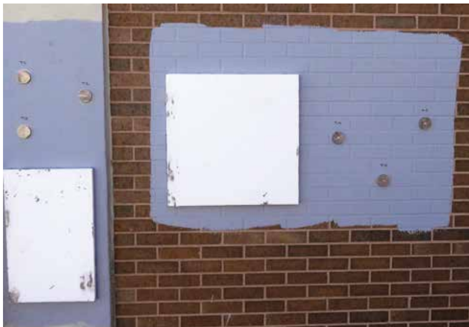
Figure 11. Mock-ups installed to evaluate adhesion of the AWB to substrates and the EIFS insulation to the AWB.
