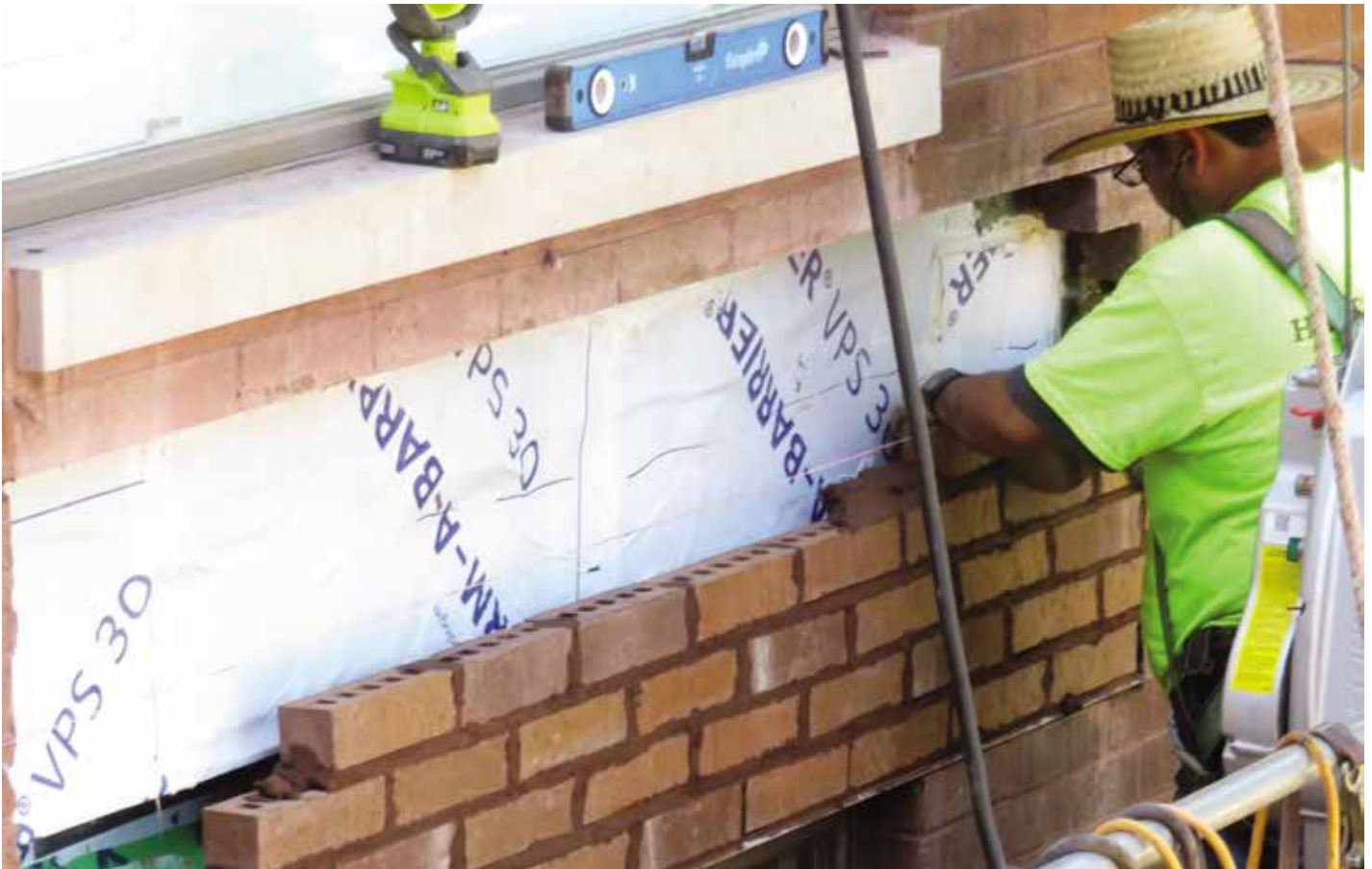
Figure 10. Installation of brick veneer following installation of the AWB and through-wall flashing.
