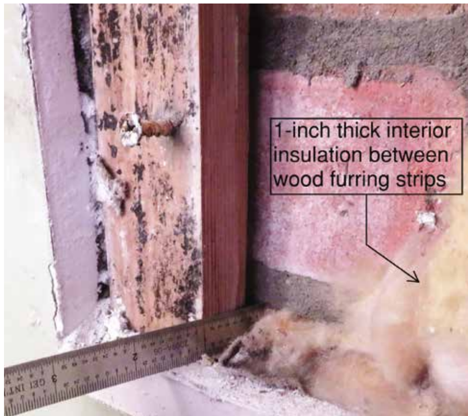
Figure 5. A thin layer of insulation provided on the interior side of a mass masonry wall.
