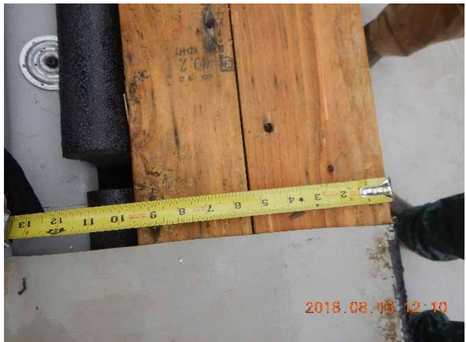
Figure 9. Top of roof curb.
