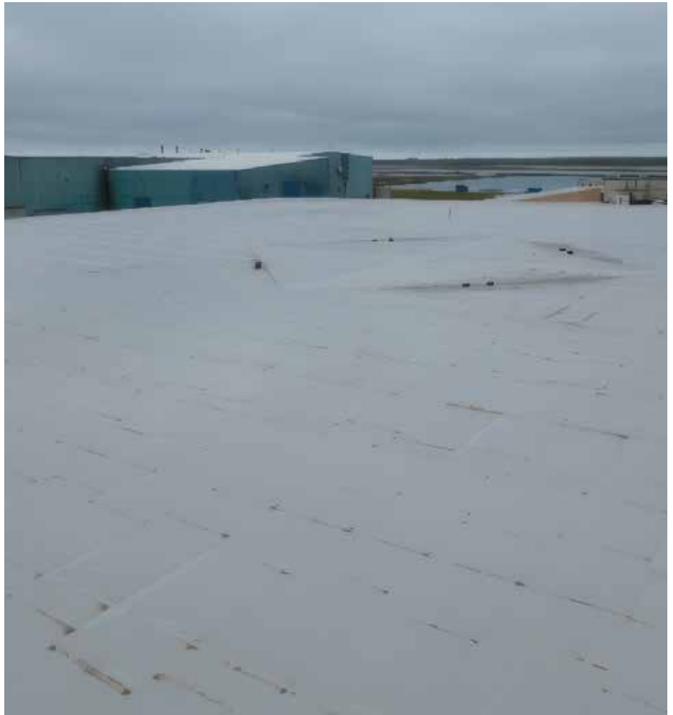
Figure 3. Overview of roof (looking northeast)
