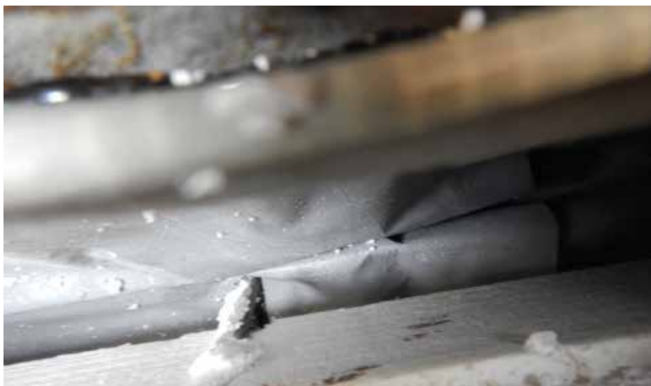
Figure 18. Close up look at the bottom of the insulation, showing more damage on the bottom layer of insulation.
