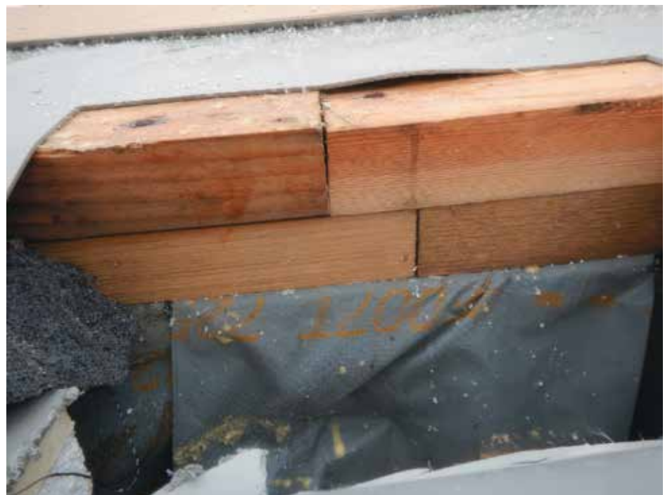
Figure 10. Built-up roof curb.
