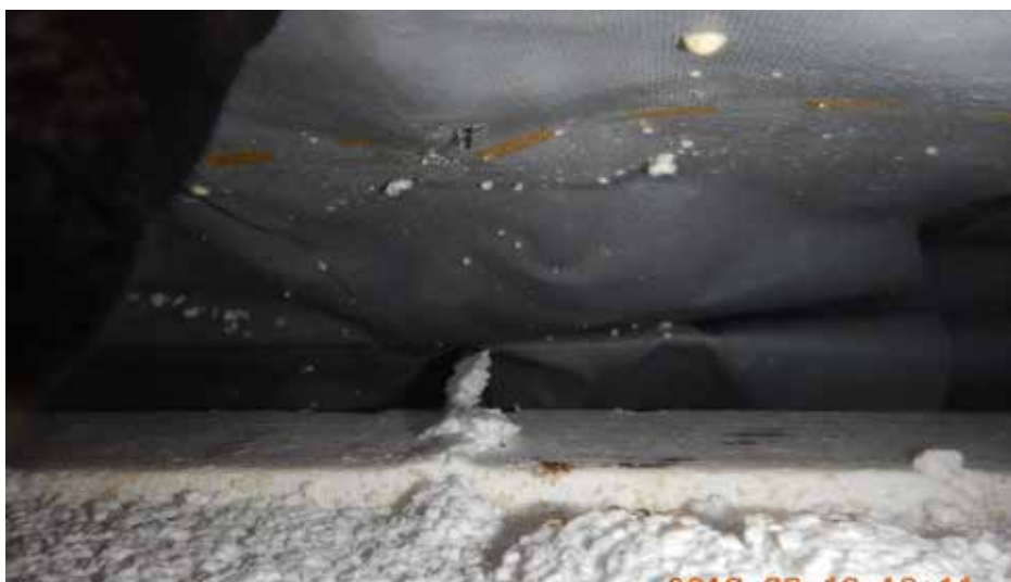
Figure 17. Downward view of rotated membrane screw tears through insulation.
