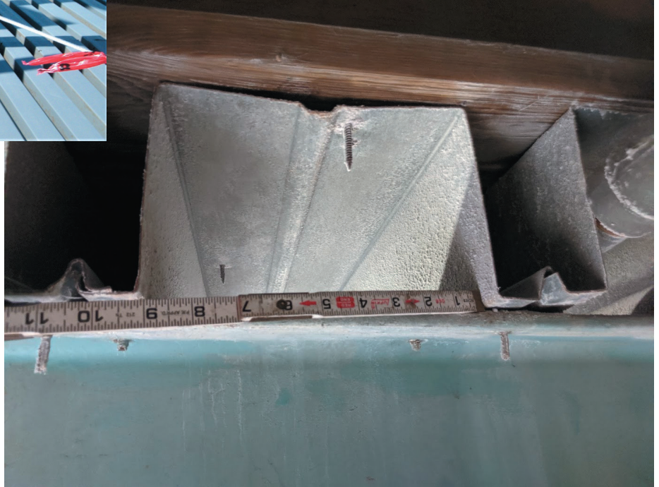
Figure 14. The 6-in. (150-mm) rib profile shown here (in a decades-old building) was not as sturdy as the profile in Fig. 13; note that the sidelaps were elevated so they could be button-punched.
