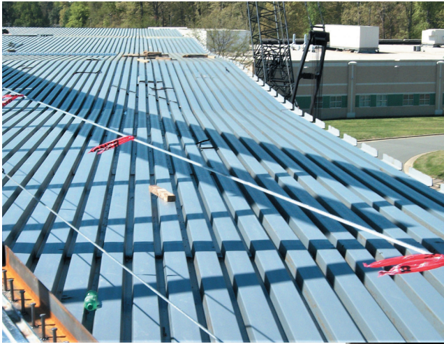
Figure 13. A 3-in. (75-mm) roof deck profile was selected for this medical testing facility. It was fastened well and was sturdy under foot.
