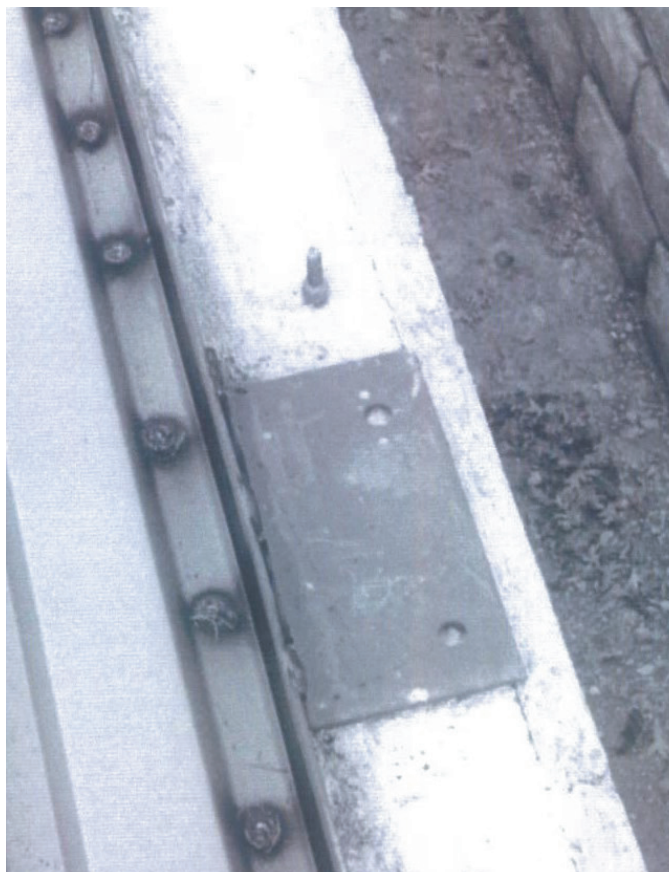
Figure 14. The 6-in. (150-mm) rib profile shown here (in a decades-old building) was not as sturdy as the profile in Fig. 13; note that the sidelaps were elevated so they could be button-punched.
