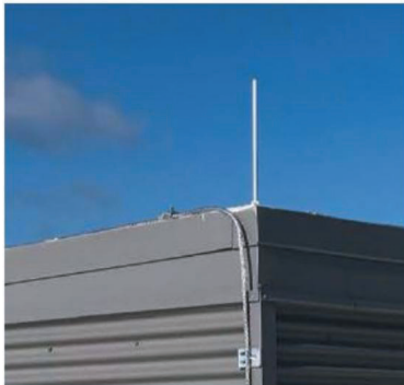
Figure 3a. Strike termination devices
