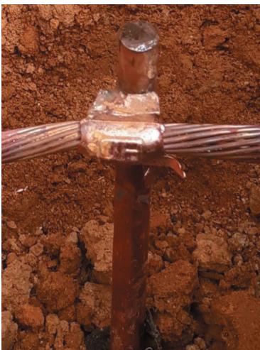
Figure 3c: Grounding electrodes
